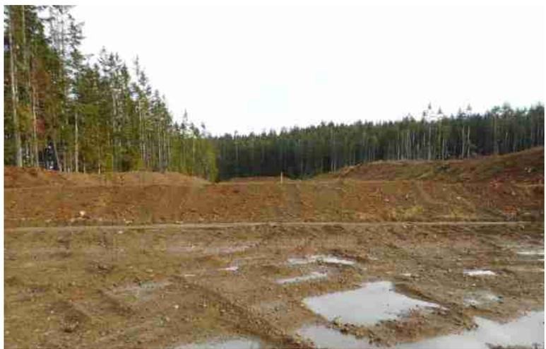
View in the the shooting direction the 6+ meter high 600 yard backstop. It reaches over the whole range including the road on the LH side
