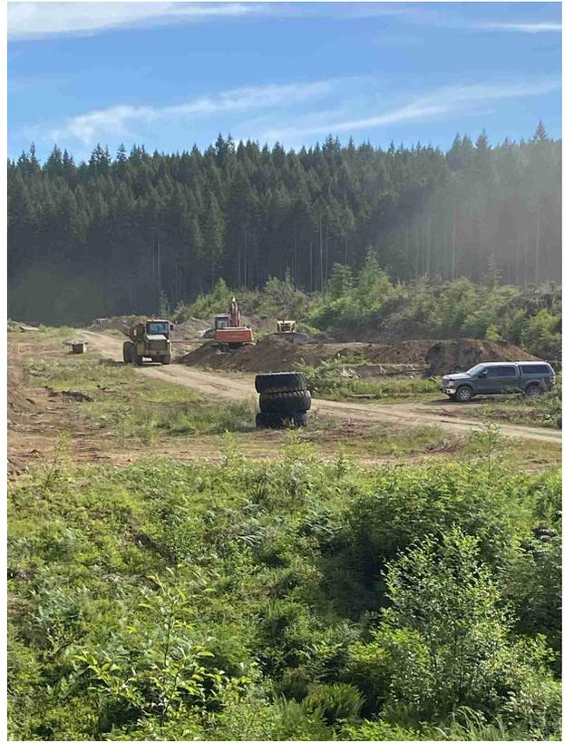
We had the use of equipment to move all the material and form the range geometry. A D6 articulated rock truck and Greg's two excavators. A 200 and a 270 Hitachi. These pictures show the range with the old road position during the transporting of material to the dynamic bays
